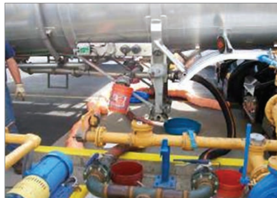
Figure 13 – Biodiesel delivery and fuel connections.
