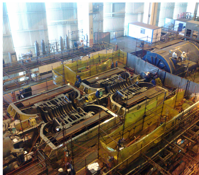
Maintenance work on LP cylinders
